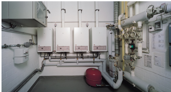
Pressure switch DL safeguards every flue gas route in the cascade
